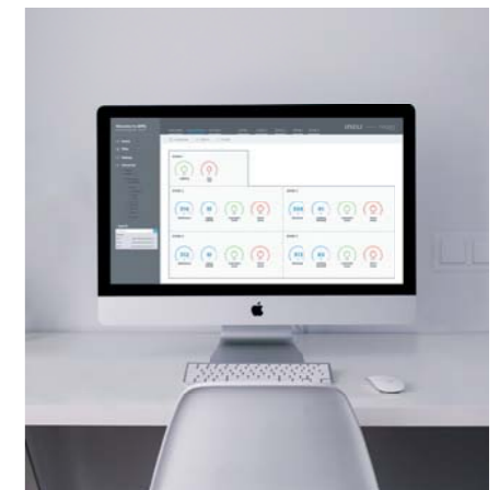
BMS (Building management system)
